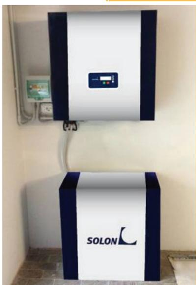
**UN IMPIANTO RESIDENZIALE DA 3,2 KWP CHE UTILIZZA MODULI E SISTEMA DI ACCUMULO FORNITI DA SOLON, STA OTTENENDO VALORI MEDI DI AUTOCONSUMO PARI ALL'80%. CON GRANDE SODDISFAZIONE DEI PROPRIETARI (E TANTI SALUTI AL CONTO ENERGIA)**
